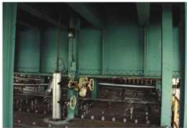
Fig. 5a (above): Thermal generation plant (fueled by natural gas). Steel overcoated with an acrylic latex. 5b (below): The coating 15 years later, maintenance free, at same location: the structure is open to a seacoast environment. Courtesy of Frank Bird, Glidden Paints and Peter Roberts, Devco Coatings
